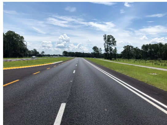
Recently completed SR-56 extension to US-301 provides continuous corridor across southern Pasco County.
